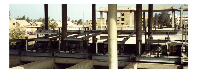
The AAF Semi-rota screen is a robust mechanically raked curved bar screen which gives a large effective screening area.
