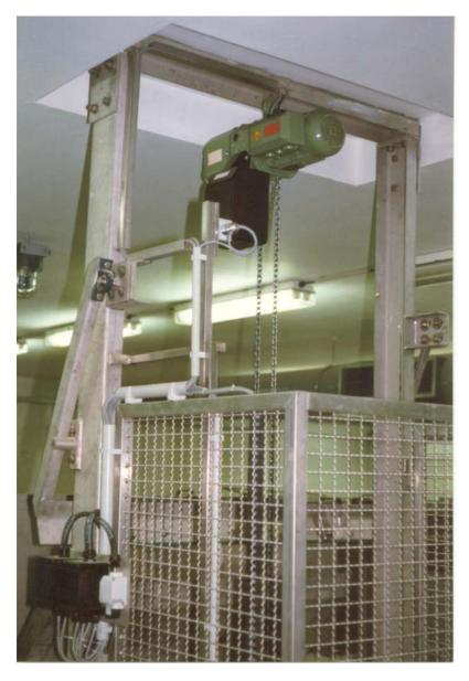
The AAF Envirotec GmbH grab type screens are designed to suit inlet channels and to protect all other equipment in the sewage treatment plant from screenings of abnormal size.
