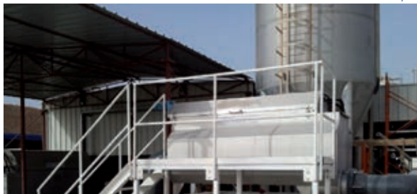
Application: Tertiary treatment, pre-filtration before Reverse Osmosis; size comparison of MSS B10-3000 in the front and the sand filter in the back, which has only one quarter of the MSS filter capacity.
