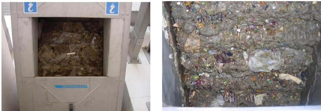
Figure 12, 13 – Proper screenings mat for a Step Screen
