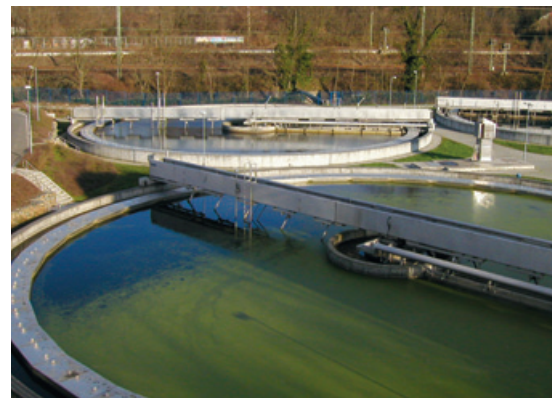
Gravity thickener in sludge treatment process
