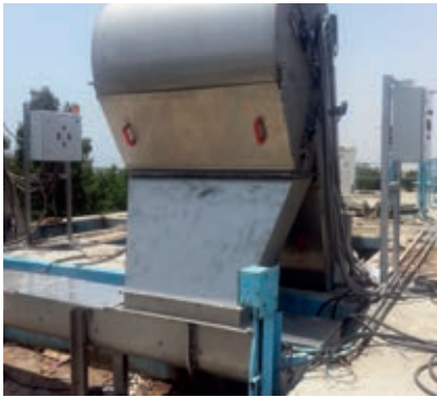
Step chain screen with screw compactor
