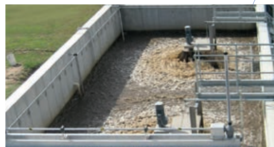
Two BIOJET™ ST 1300 with the unique one cell floating construction in a rectangular tank
